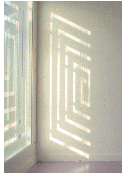
Below: Martin Richman, Jubilee School, Tulse Hill, London 2002. Photo: Tim Soar. Richman devised a spiral pattern which was sandblasted onto two sheets of glass for an external window at the end of the first floor corridor. The double layered pattern created an interlinking screen to obscure direct vision to nearby buildings whilst still allowing sunlight into the corridor.
